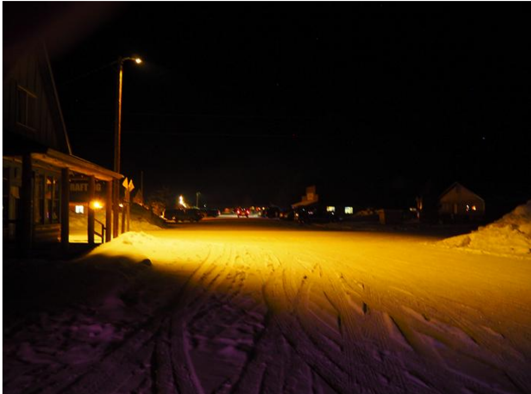
Figure 21: Lumicana, 60-80 Watts, LED, shielded, 2200 Kelvin, 8400-11,200 lumens, in Stanley, Idaho. (Different wattage and lumens were used for different intersections). Installed in 2019. Photo: Mayor of Stanley.
