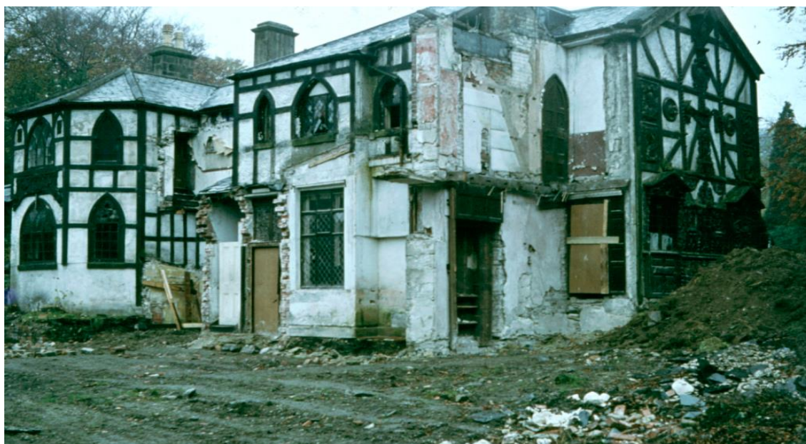
Figure 3 removal of extension, Llangollen Museum 2012
