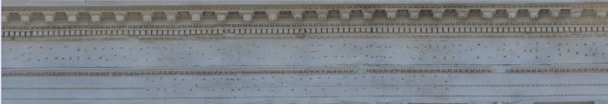
Figure 3 —inscription holes- http://www.maisoncarree.eu/monument/architecture/facade-principale/dedicate
