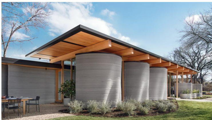
ICON and Lake Flato build 3D-printed House Zero in Austin (2022), [photograph] (Accessed: 9th May 2022)
