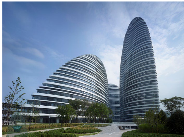
Figure 29: Zaha Hadid, Wangjing SOHO building in Beijing (Photo credit: V. Bertrand)
