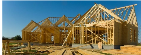
Figure 20: The construction of a dwelling (Photo credit: H&H Builders Inc)
