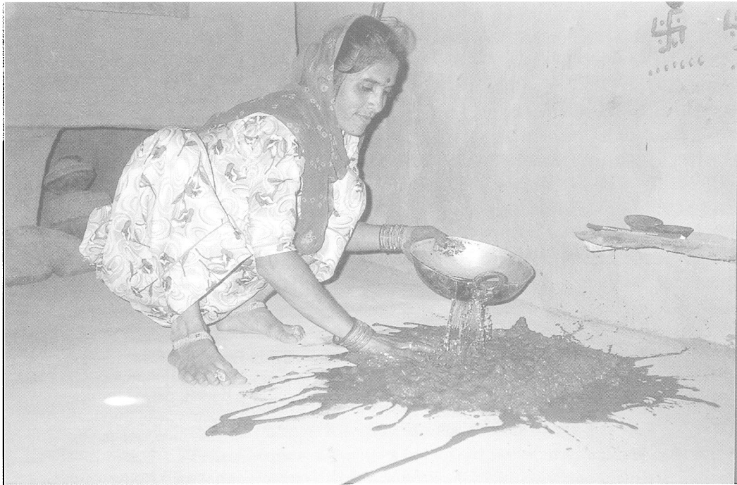
Plate 1 A Rajasthani village woman replastering the floor of her house in preparation for a ritual that will be held in the house later on in the day (see Plate 2). The plaster contains cow dung, water and a type of red soil called pili mitti or Laksmi mitti .
