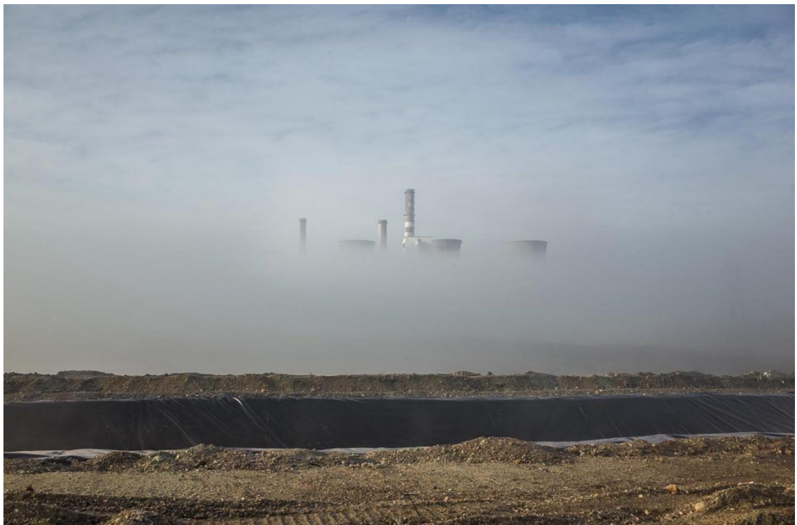
Fig 1: Fog shrouds a power plant in Ptolemaida, in northern Greece
