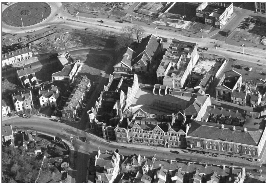
Aerial view of bomb damage at Dynevor School in aftermath of World War II.
