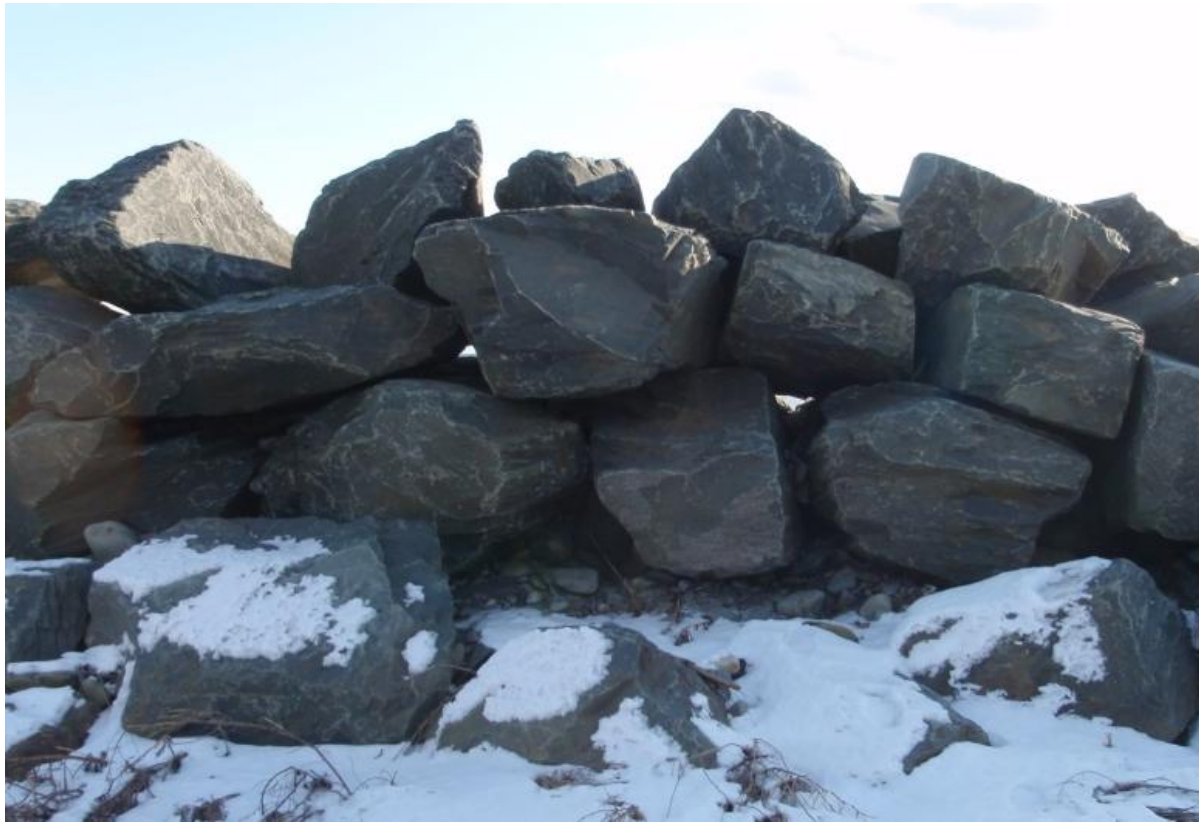
Figure 1 Armour layer of Cow Bay causeway revetment
