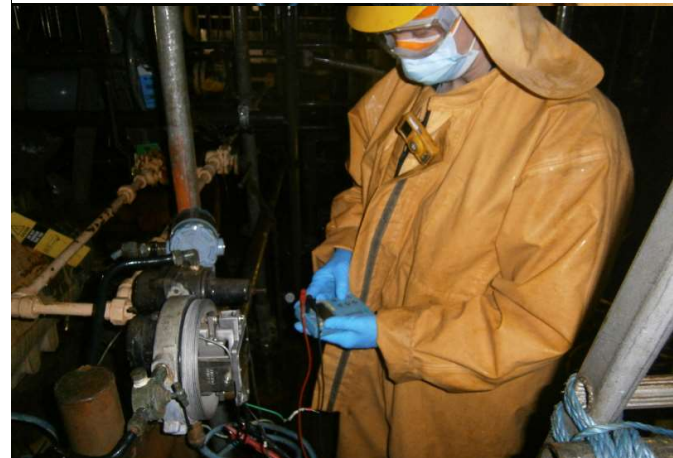
Figure 4 Connecting mA source
