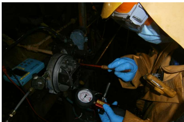
Figure 7 Adjusting zero point
