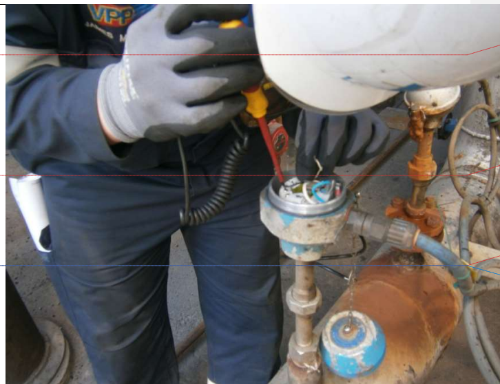
Figure 10 Reconnect thermocouple to transmitter
