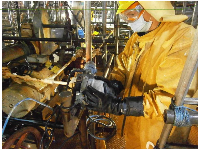
Figure 2 Removing instrument cover
