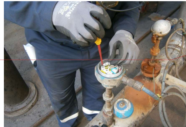
Figure 2 Disconnecting thermocouple from transmitter
