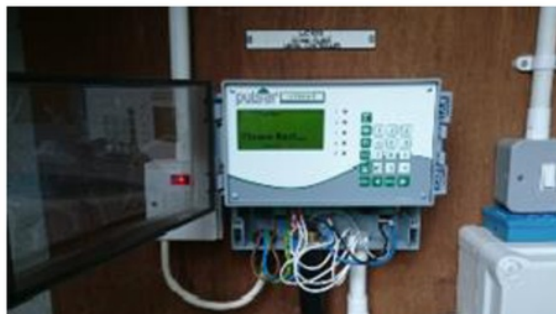
Figure 19: Connection of the Level Controller to a 240V supply, fixing it to the wall and connecting the ultrasonic head to the controller.
