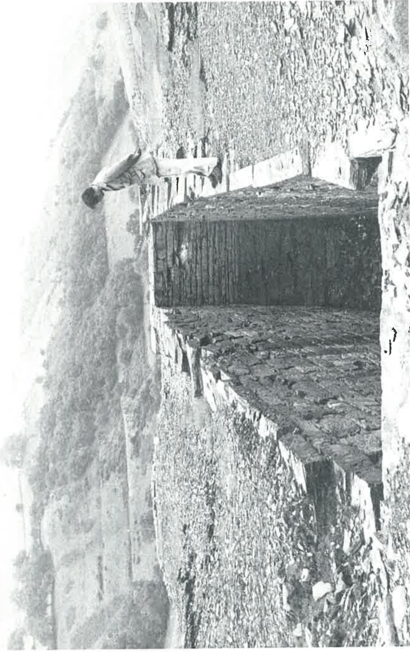
PLATE VI The pit for the 56ft. waterwheel at Wemyss, used for pumping Frongoch via flat rods. (R.H. Bird)
