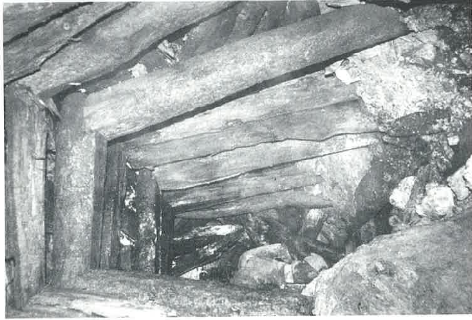
PLATE IV. In the Frongoch Adit 1986: timbering in soft ground. (S. Timberlake)
