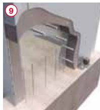
Rebar set into foundation (by others), centered between Bi-Steel connecting bars
