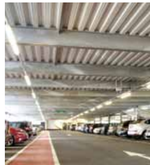
Comflor 80 with Colorcoat coated underside
