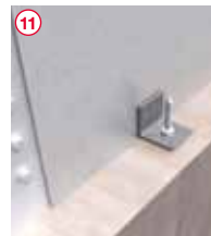
Angle welded to Bi-Steel panel to accept temporary holding down bolts cast into the foundation
