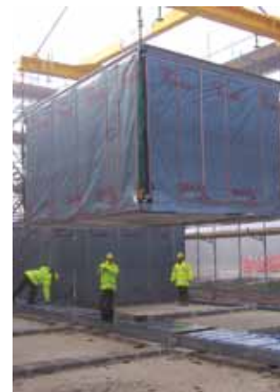
Build process on-site
