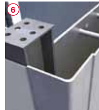
Pressed angle welded to 2 Bi-Steel panels to form corner module
