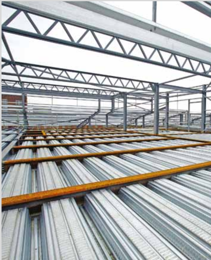
Slimdek flooring system at St Richard's Hospital, Chichester
