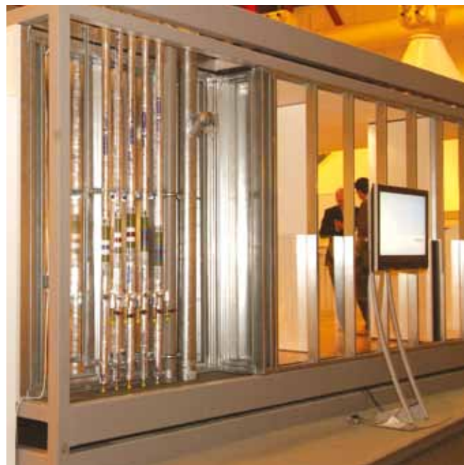
Layout of vertical riser
