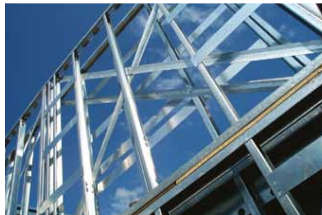
Structural cold formed sections in use
