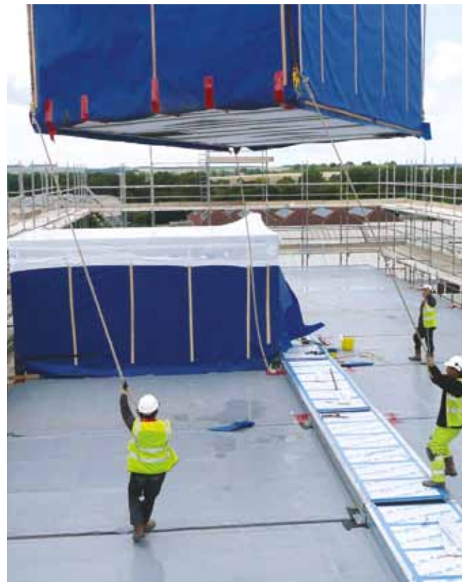
The on-site build process
