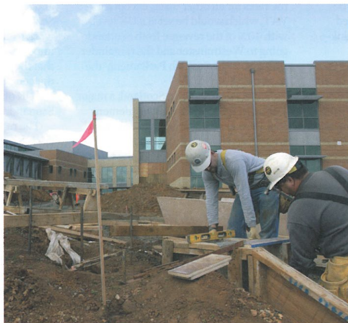
Laying the foundations: the Private Finance Initiative is popular for school rebuilding
