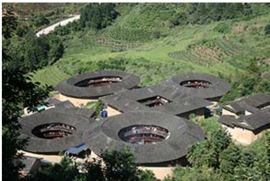
Figure 3.3. Tianluokeng Tulou Cluster. This view of the five buildings shows how the site can be articulated as an example of architecture-nature harmony.
