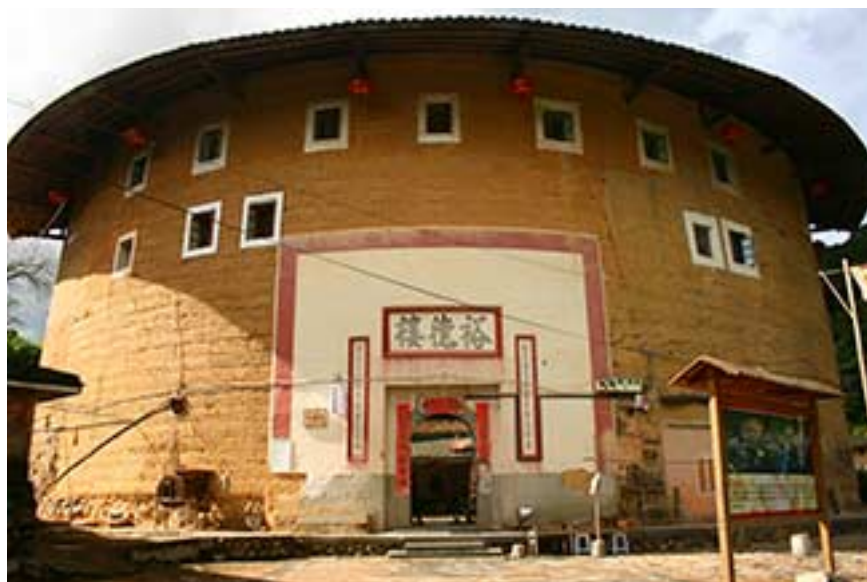
Figure 3.1. Exterior of Yude Lou, a designated building
