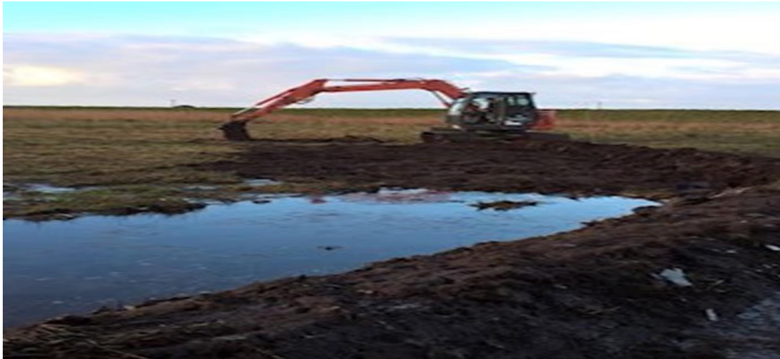
Fig 4: Photograph: depicting low pressure bund reprofiling at Cors Caron NNR from 'Life for Welsh Bogs Blog'(2022)
