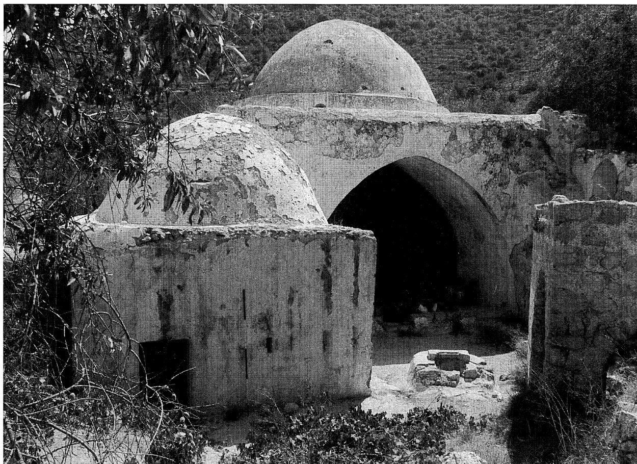
Figure 2. General view of Dayr al-Shaykh with large dome of prayer hall and smaller dome of the maqam.
