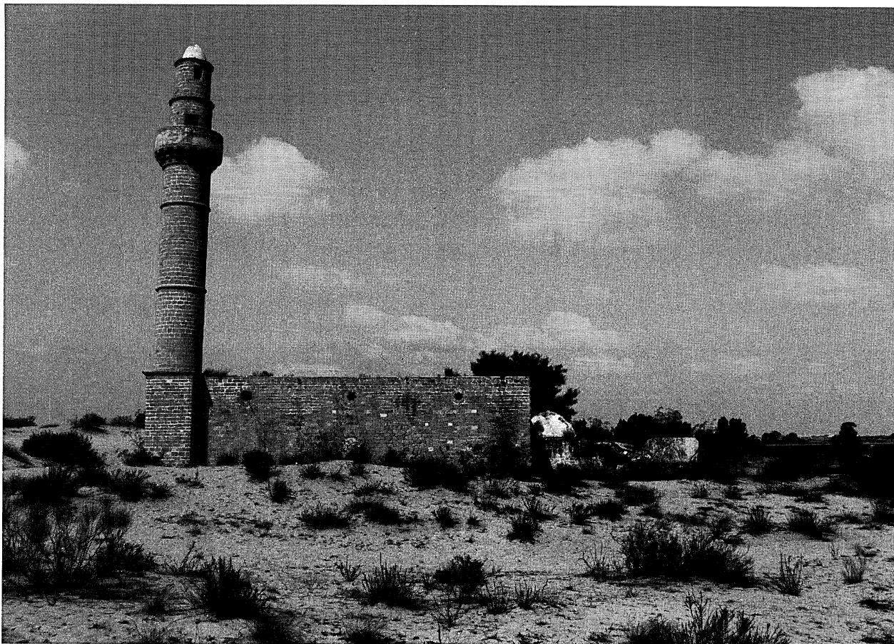
Figure 6. Nabi Rubin, general view from the south before the destruction of the minaret in 1993.
