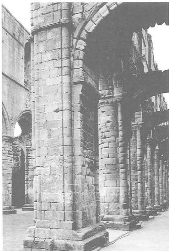
Fig. 5. Fountains Abbey, north-west crossing pier, detail from north-east. (author)
