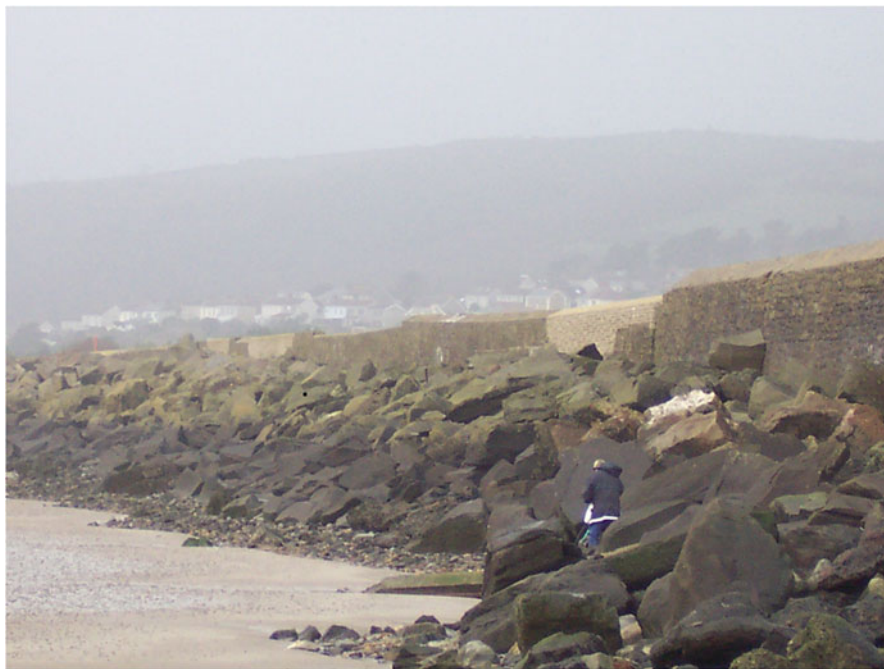
Fig. 17.12 Rock armour protection of rail link
