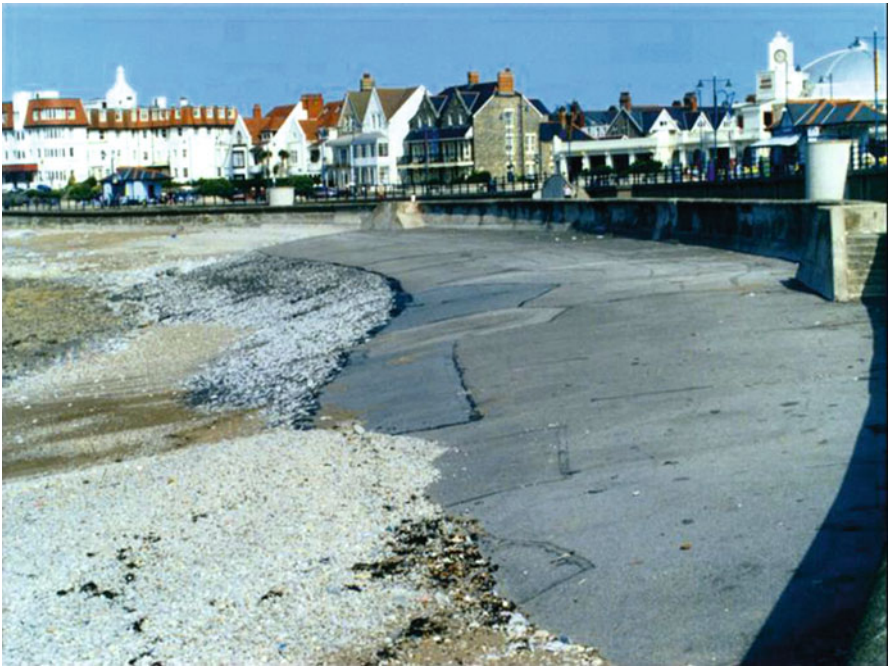
Fig. 17.5 Bitumen revetment covering upper beach
