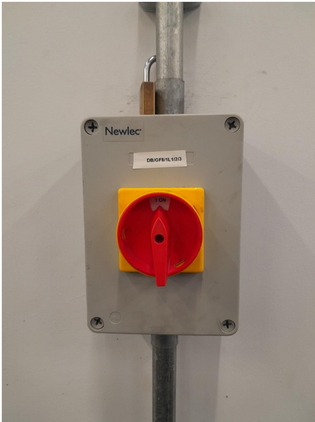
Figure 13: Lathe emergency stop switch.
