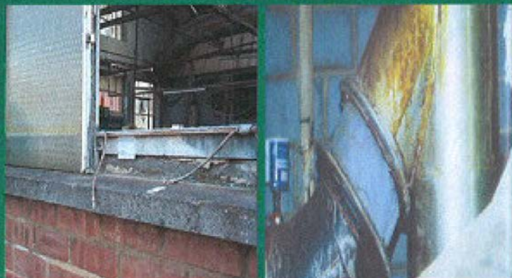
Packing to window frame
