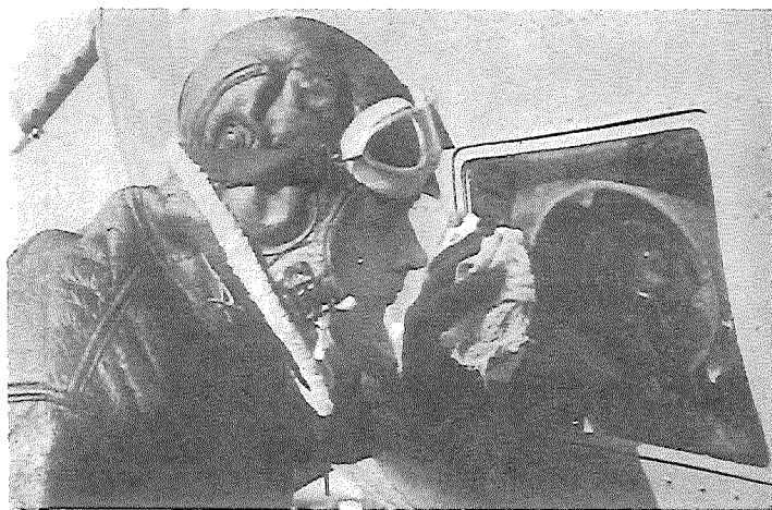
35. Cameraman cleaning the glass lens-cover of a Trimet' sloping camera on board a B-17.
