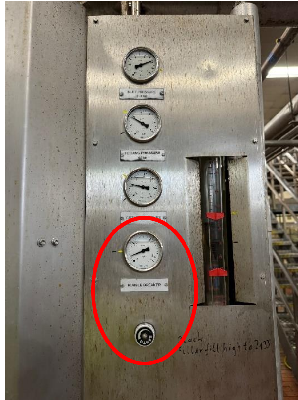
Figure 3 – Adjusting Bubble Breaker Regulation of CO2 Pressure
