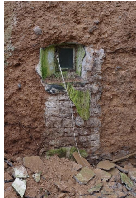
Figure 2 Blocked door opening in the north elevation after the removal of the render © Cornwall Council.
