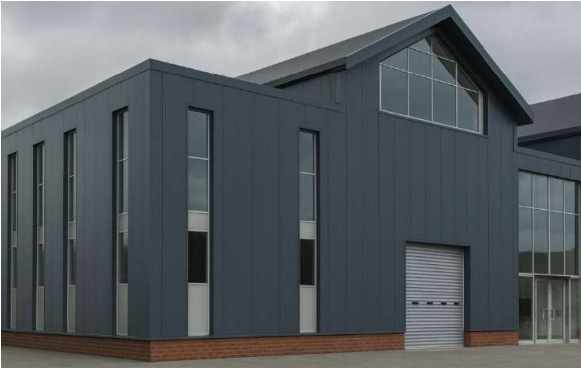
Image 14 - South-East Exterior View (OpenAI, 2026b)
