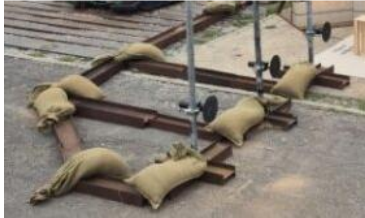
Figure 4 – Pressure Gauges and Cable protection
