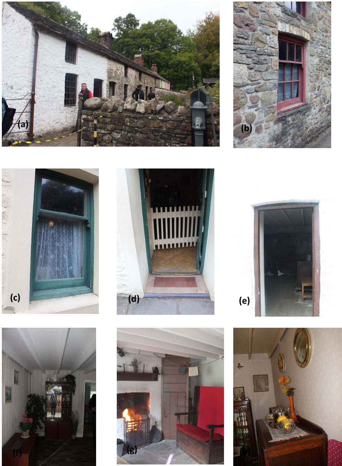
Figure A1: External view of terrace houses (a), Interior wall finishes (early period). Sub-figures (a–h)
