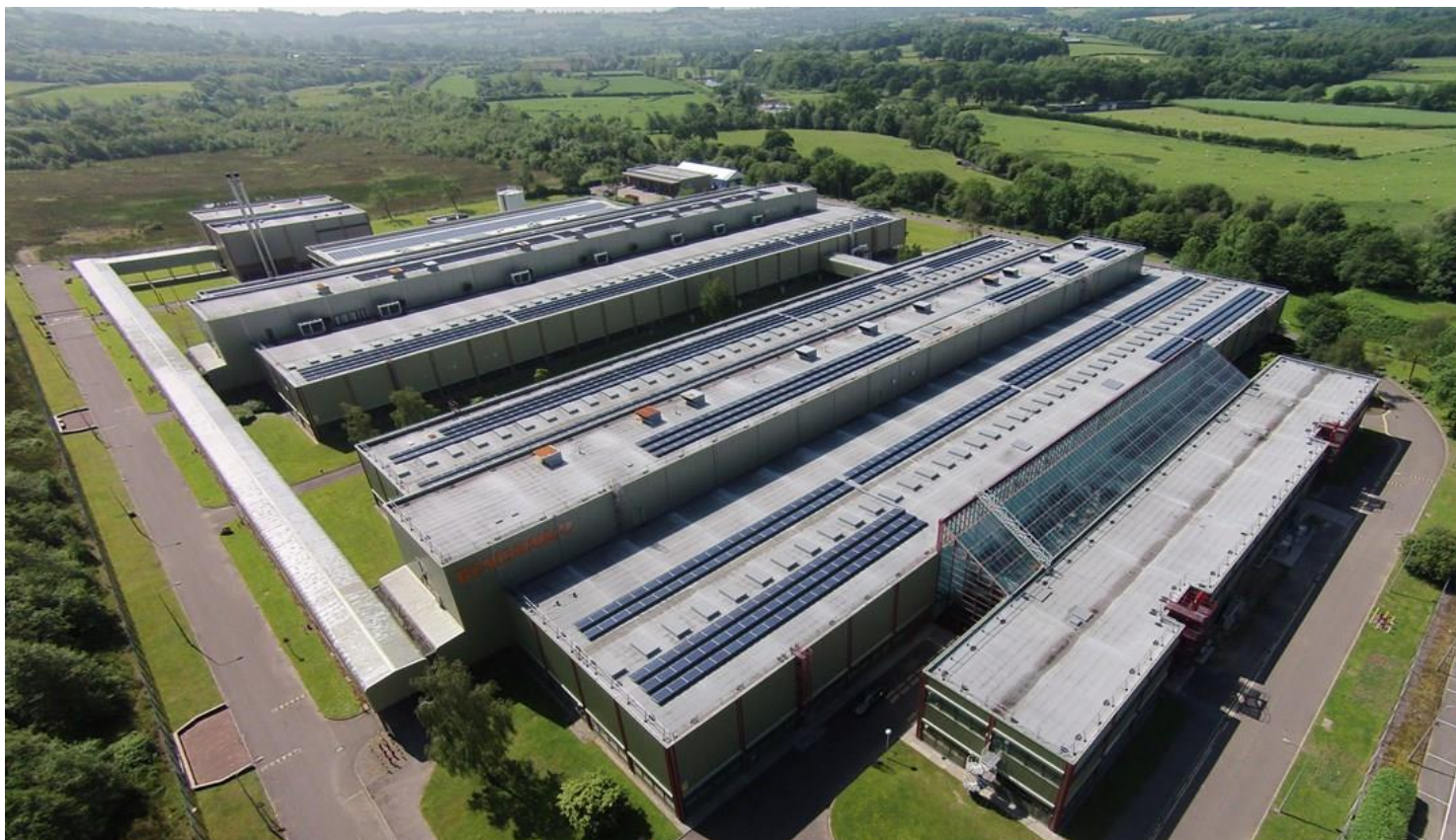
Renishaw Miskin Site - Photo reproduced from [1]
