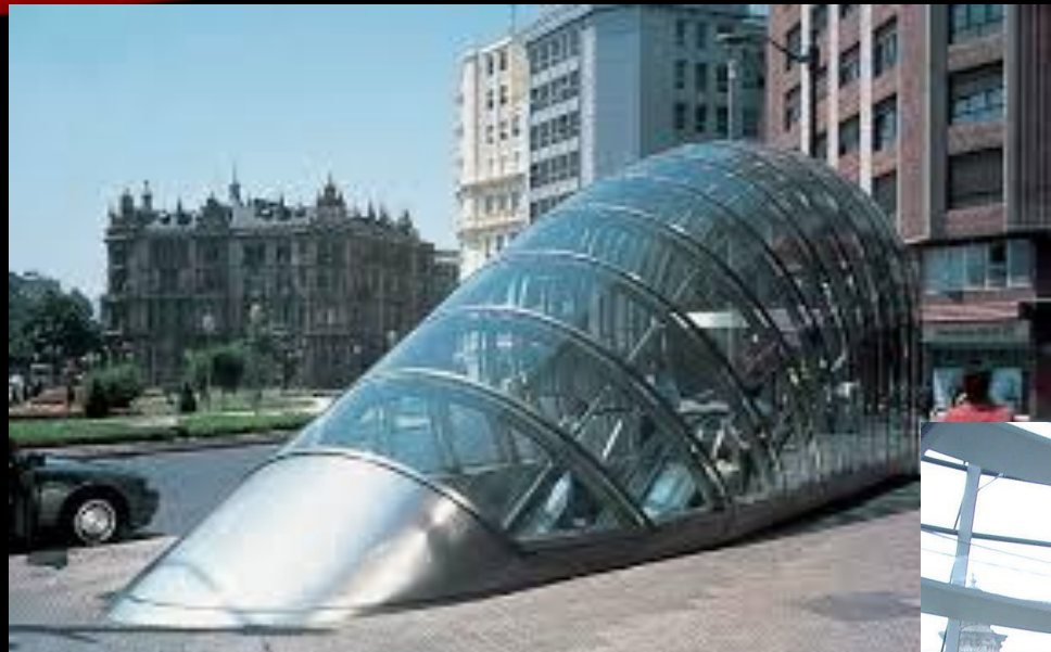
Metro Bilbao Station (1995)
