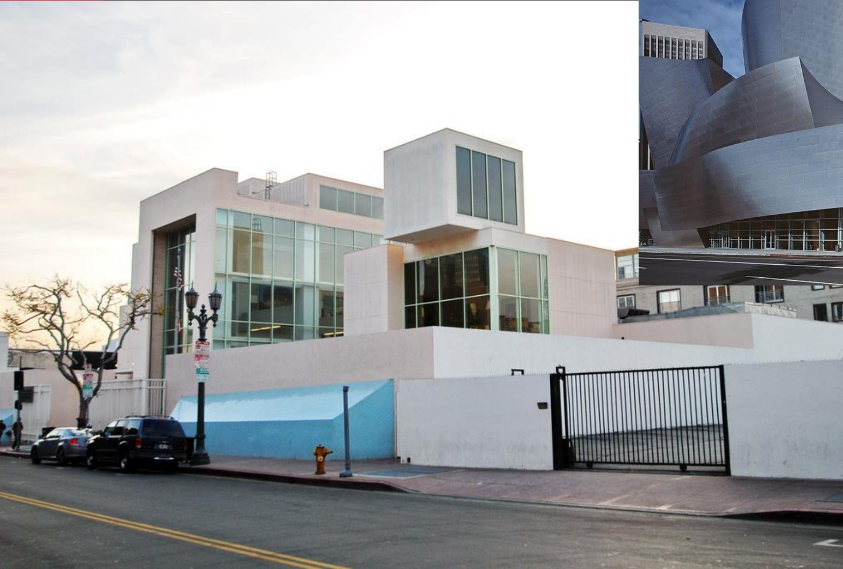
Frances Howard Goldwyn Hollywood Regional Branch Library Designed by Frank Gehry (1986)
