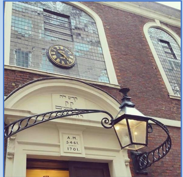
Figure 10 – Entrance of the Synagogue
