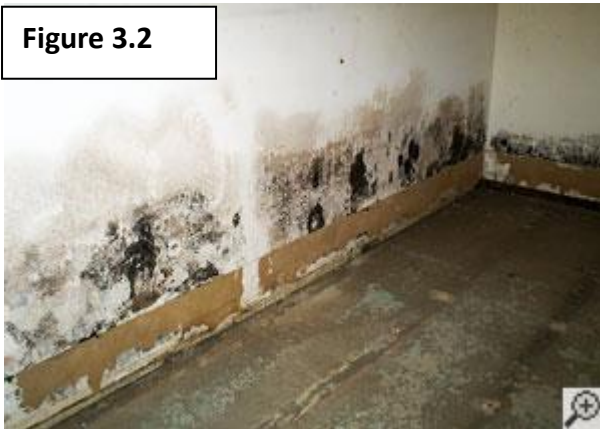
Figure 3.2 – Mould Damage
