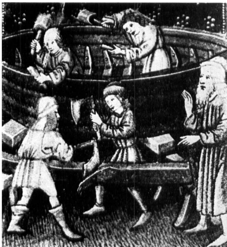
Figure 19. Boat built by "shell" technique in the 15th century. The planks are probably fixed to one another by clamps; the dowels fixing the floor-timbers are driven in with mallets. (After Moll, 1929, G 1, c 13.)
