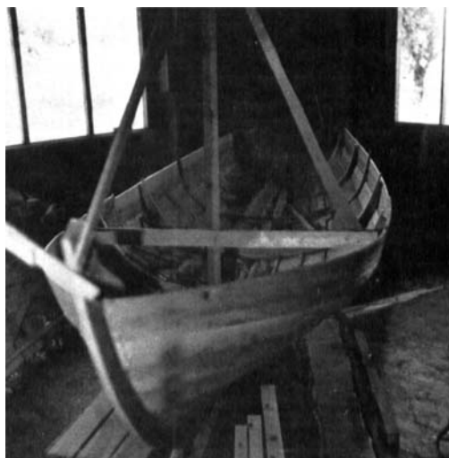
Figure 23. Clinker-built boat under construction, western Norway. The mould of which only the upper part is visible, is still in place at the last stage of building. This type of mould is in the form of an arc of which the extremities are joined by a cross-piece. (Photo by courtesy of A. Thowsen, Director, Bergens Sjøfartsmuseum.)
