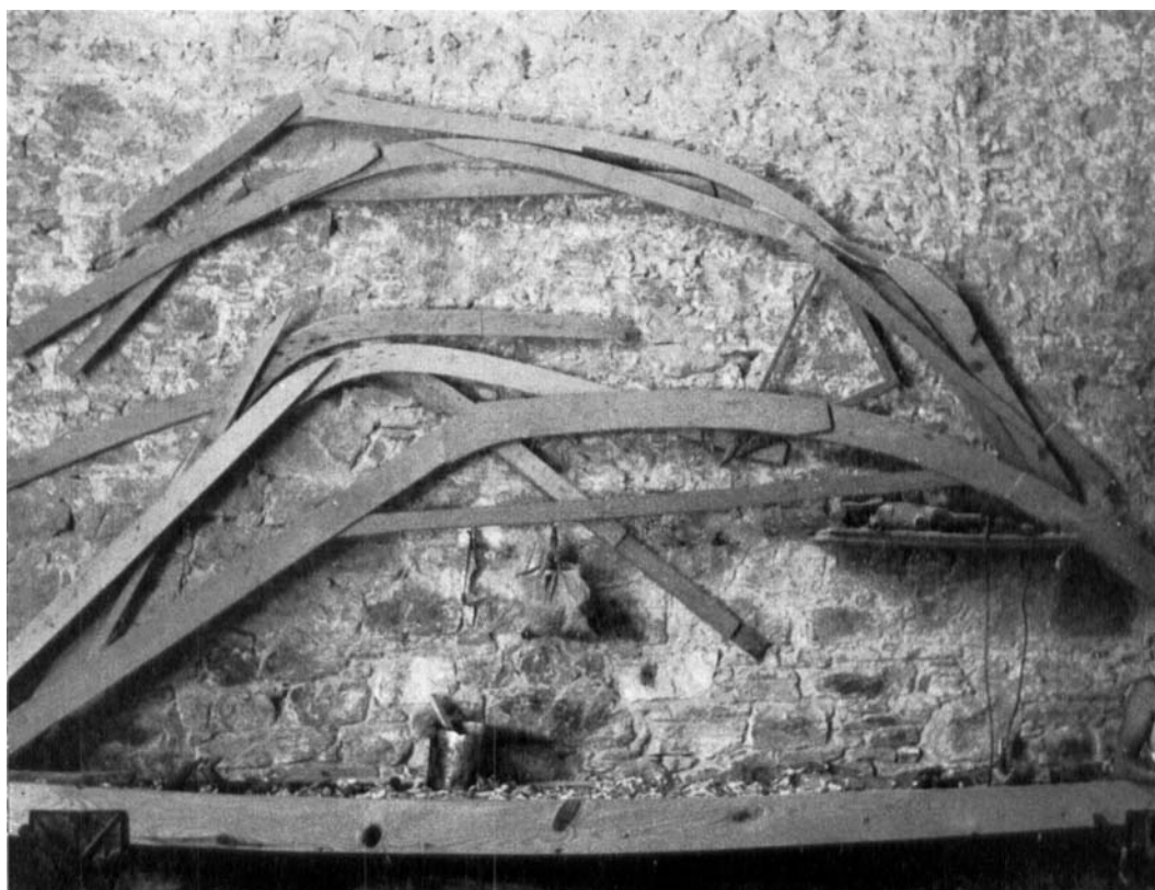
Figure 24. Templates used in a Syra boat shed (Syros). These moulds contrary to those shown in Figs 23 and 26 are not intended for erection on the keel, but to establish the shape of the more important structures of the ship, the frames as well as the stem and sternposts. (Author's photo, June 1969.)
