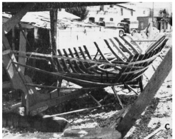
Figure 25. Shipyard at Marathokampos, Samos, June 1969. The form of the central frame has been established by a mould. The provisional battens serve, so far as the shape of the intermediate frames is concerned, exactly the same purpose as the planking in "shell" technique. (Author's photo.)
