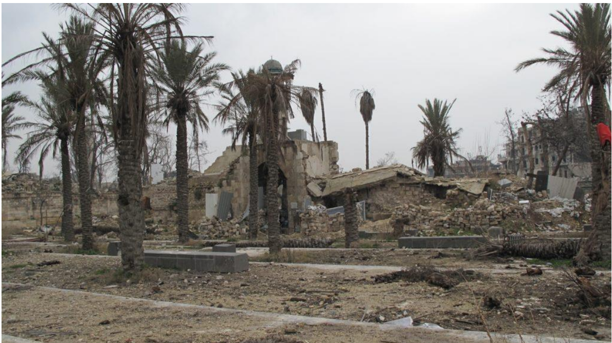
Fig 15: The destruction of Al Sultania Mosque, Aleppo's Old City (Buffenstein 2017).
