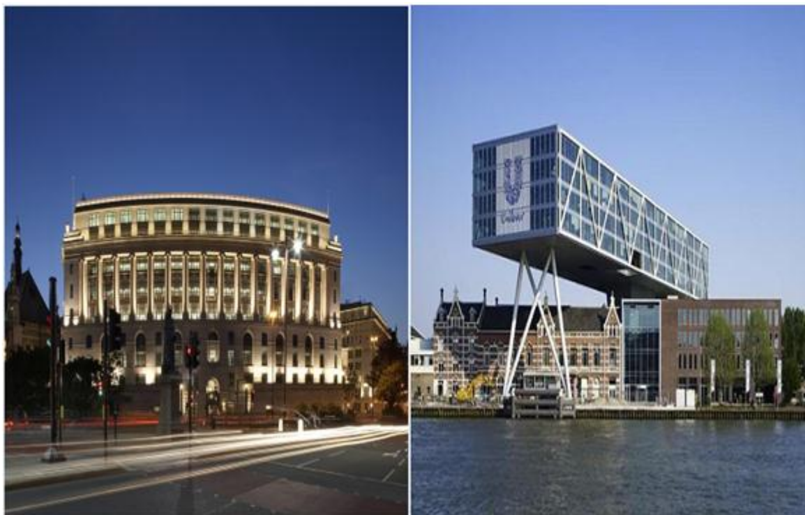
Figure 1: Unilever's London and Rotterdam headquarters
