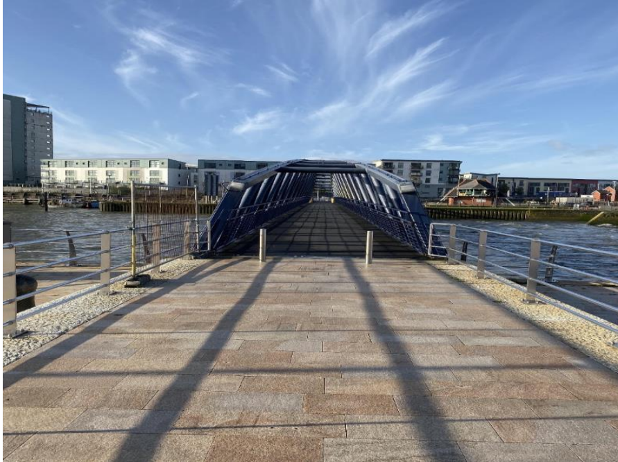
Fig 2: Picture of Swansea's arch bridge in SA1
