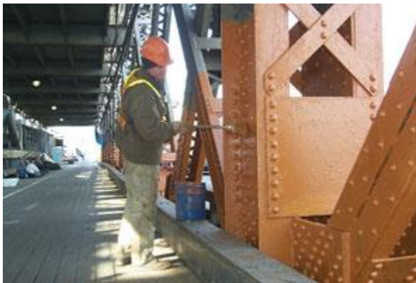
Fig 5: copper paint for a steel bridge.
