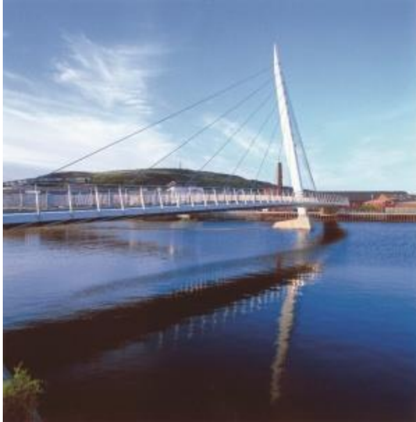
Fig 3: Swansea's simple but aesthetically pleasing sail bridge
