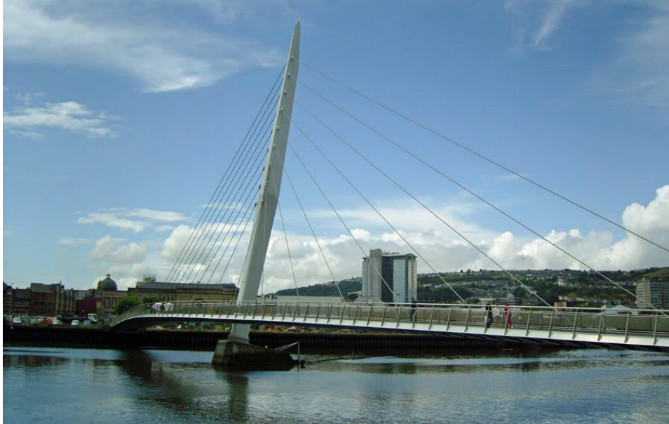
Fig 4: Swansea's steel deck sail bridge
