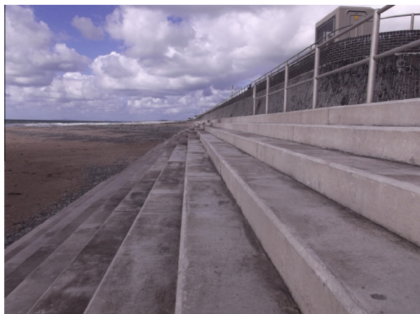
Fig. 2a. Towyn, an old fashioned resort with a new Sterling £11 million seawall.
