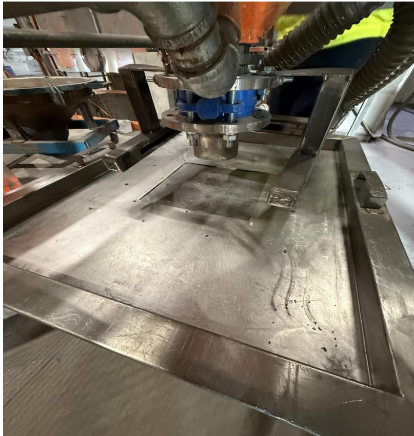
Figure 10 – POD Decant station with oversize grill and extraction unit fitted.
