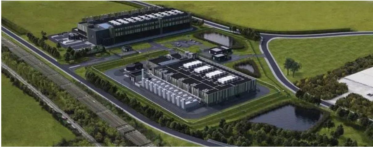
Figure 8: AWS data centre in Didcot
