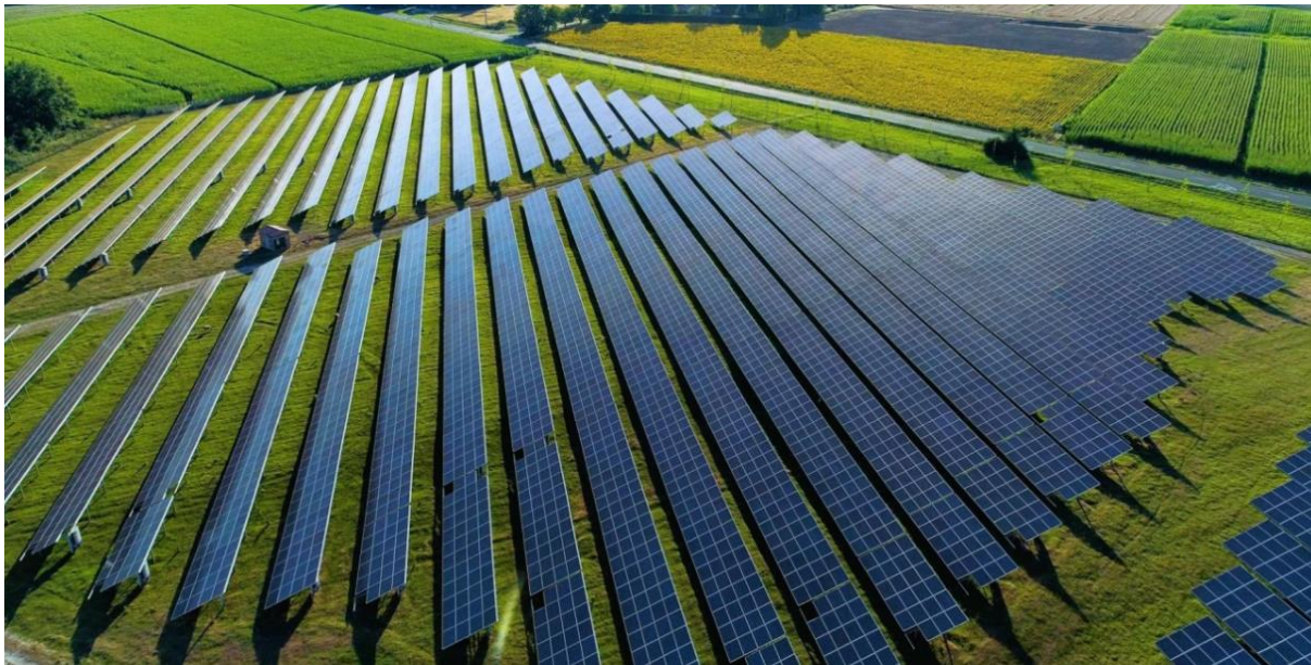
Figure 15: AWS solar farm
