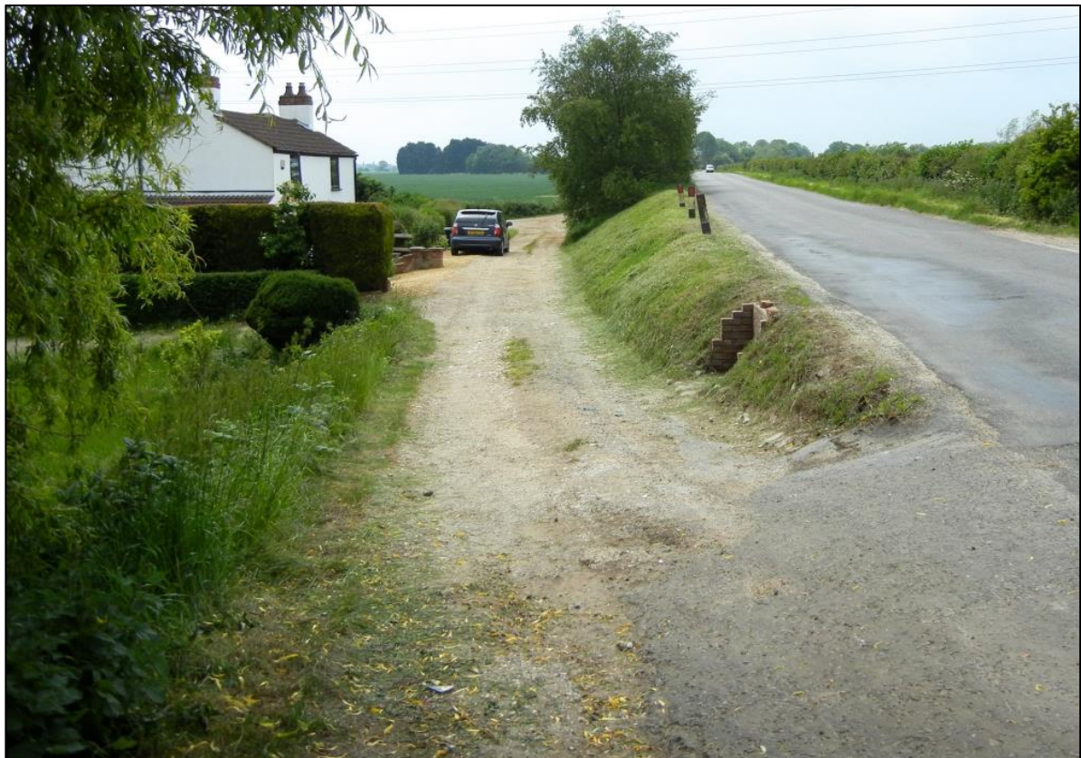
Plate 1.2: View to the west along the extant Sea Bank near Walpole St. Peter (Oosthuizen 2016)
