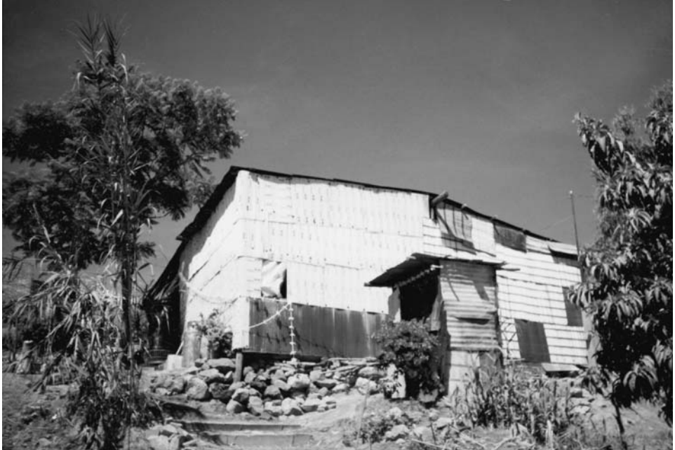
Plate 4.1 Self-built house, informal settlement, Oaxaca City, Mexico.
