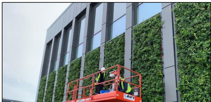
Figure 6: Preservation contractor Biotecture LTD using a scissor lift to perform maintenance on the MLWS at IMPACT (Author, 2019).
