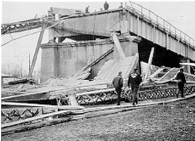
Figure 10: Collapsed silver bridge in West Virginia (1967) collapsed in less than a minute killing 46 people
