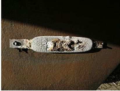
Figure 20: Sacrificial anode attached to prevent corrosion (Gretchen, 2015)
