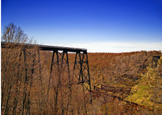
Figure 11: Collapsed Kinzua Bridge in Pennsylvania was blown away by a tornado since its central bolts had been eaten away by rust leaving the bridge anchored by gravity
