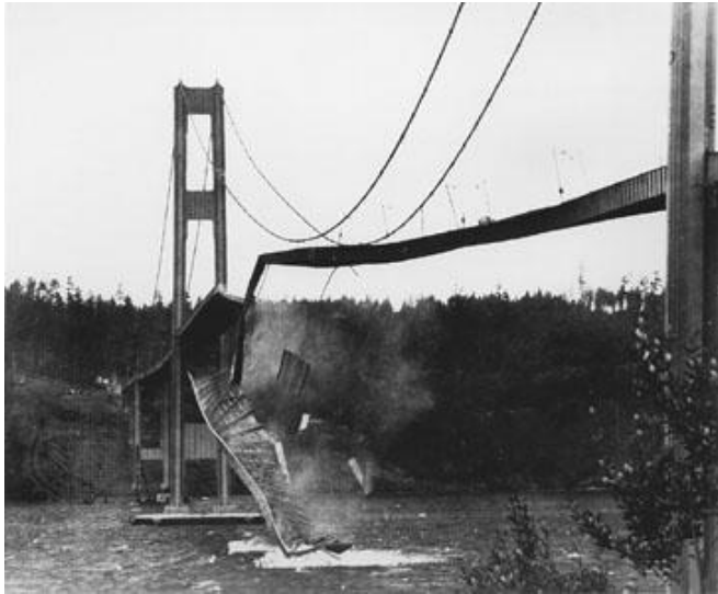
Figure 1 Tacoma Bridge Collapse due to Simple Harmonic Motion (SHO) (Study.com, 2022)
