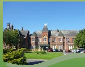
The Learning and Development Centre at Duncan Macmillan House, Nottingham
