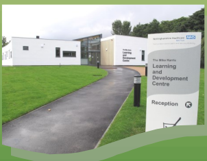
The Mike Harris Learning and Development Centre at Rampton Hospital
