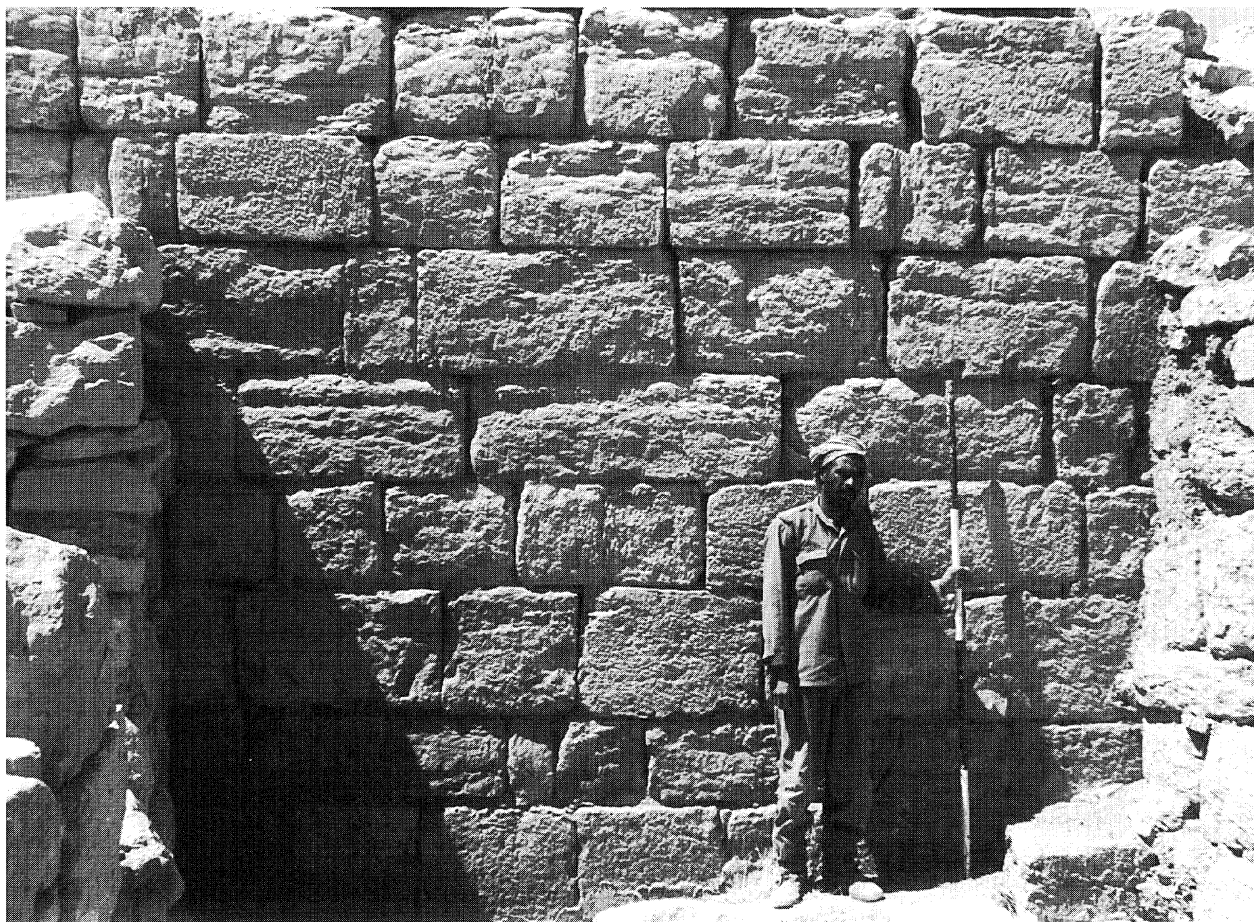
Figure 5. The northern façade of the north wall of the Double Enclosure as viewed from within the church, with a later Islamic wall abutting to the left.
