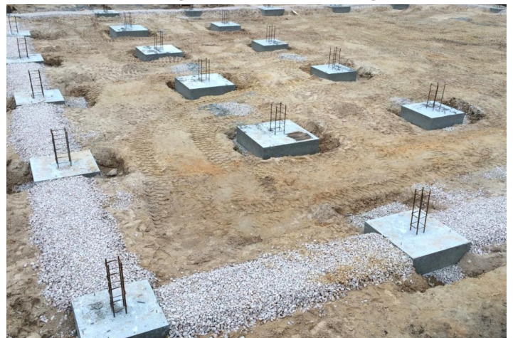
Figure 7 www.iss.lv . (n.d.). pad foundation construction. [online]
