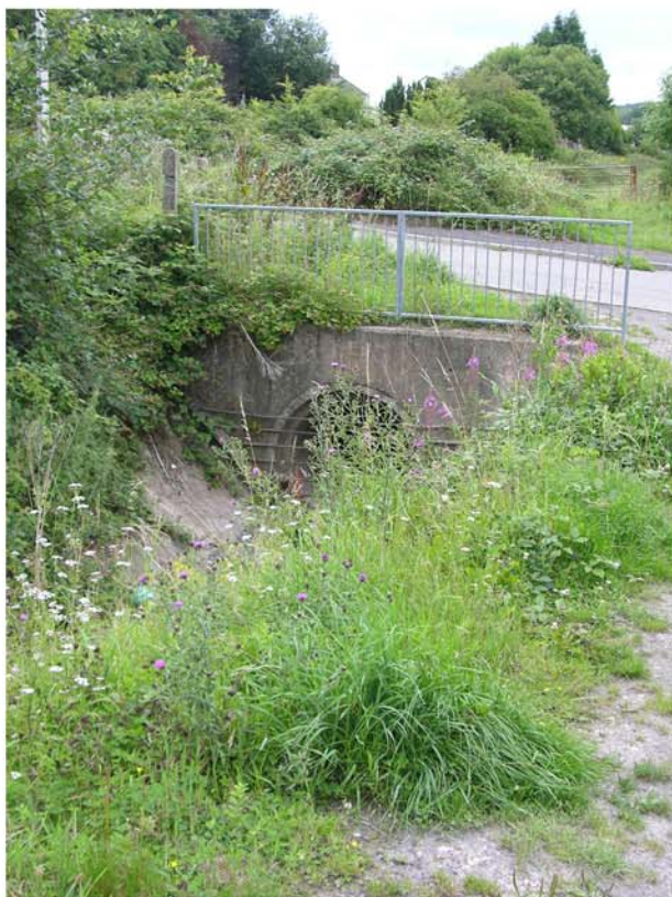
Culvert at north eastern corner of the site.
