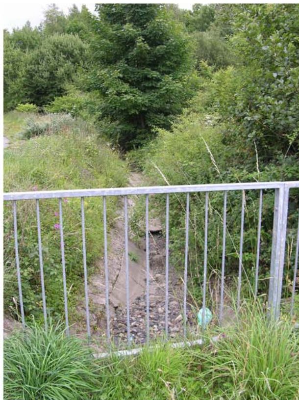
Watercourse at western boundary.
