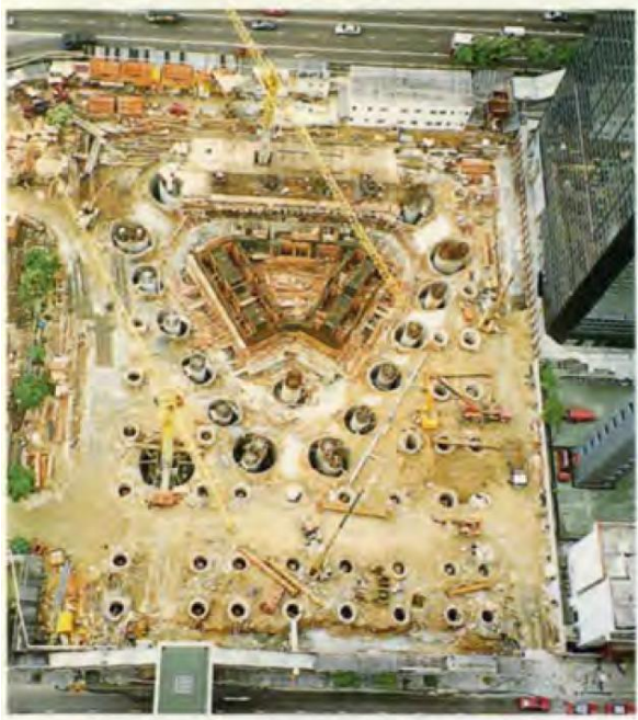
Figure 4: Foundations from the air, showing the very large diameter main caissons. (Ayres and MacArthur, 1993, p. 19)
