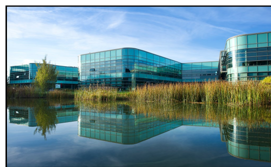
Figure 5: Faculty of Health building (Edge Hill University, 2017).
