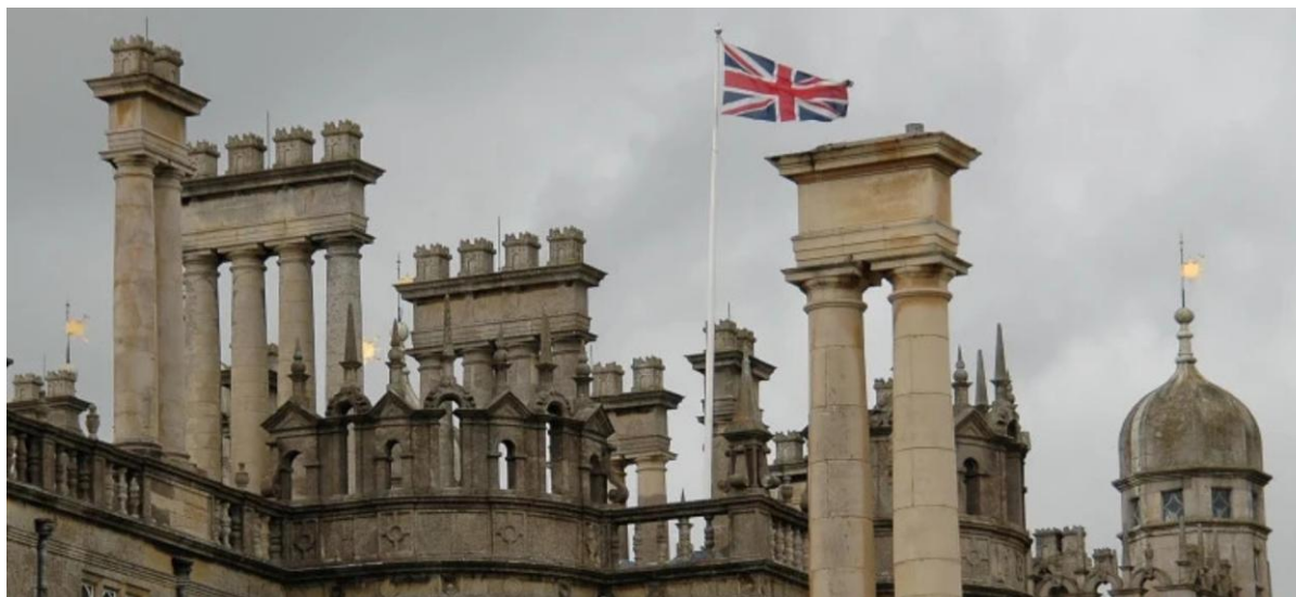
Fig. 11 – Burghley House chimneys. (Montacute Pavillion, 2014)
